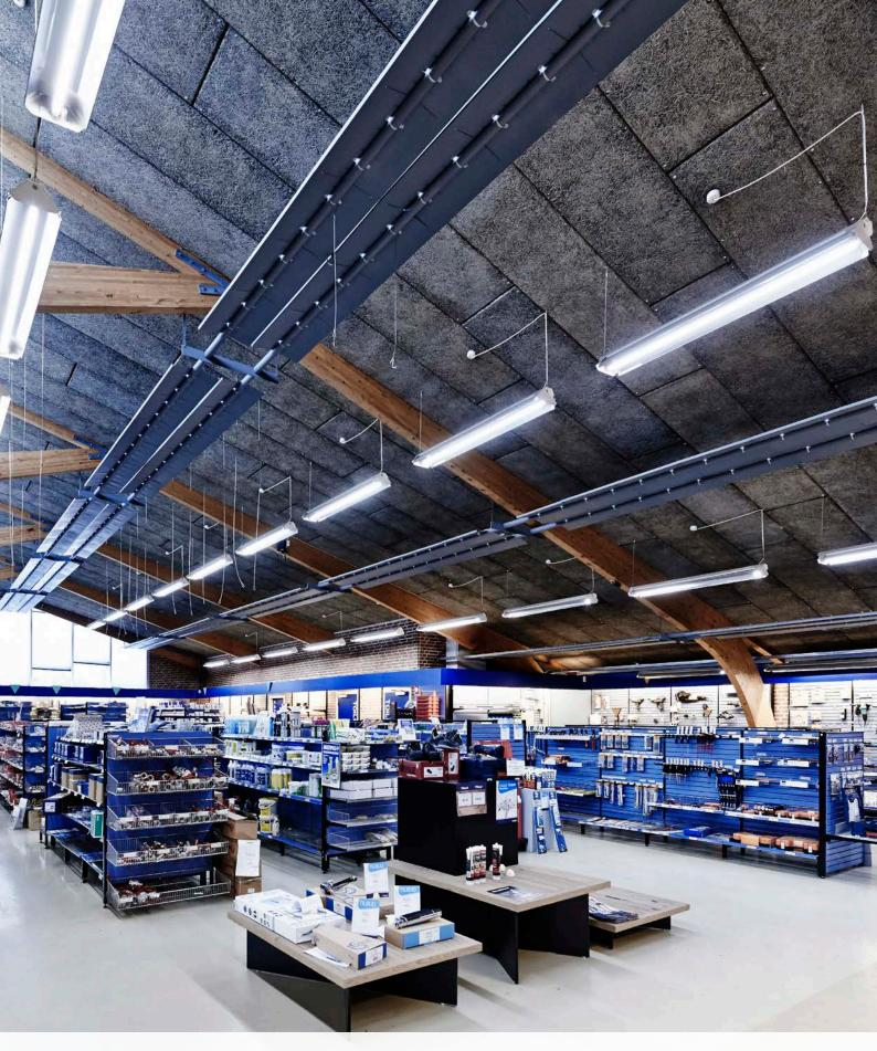
In 2013, a pilot project was launched in Sanistål's outlets in Aars and Aalborg as these outlets' working environment was affected by excessive heat in the outlets during the summer. All luminaires were replaced by energy-efficient LED lamps and the roofs of the outlets were painted with a special reflective paint.
