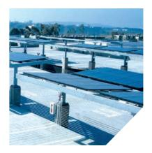
Over 2,766 photovoltaic solar modules sit atop roofs and carports at Qualcomm's San Diego campuses, providing the Company with 500 kilowatts of power.
