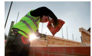
In 2013, toolbox talks have been delivered relating to scaffold use and internal fall protection/prevention
