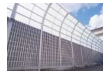
Dai Nippon Printing Technopack Kansai Kyoto plant: Sound-proof wall
